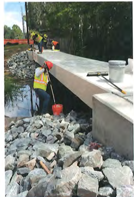
Pine Avenue Sidewalk Improvements
